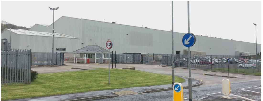
The former Caterpillar Factory on Doagh Road, Monkstown
