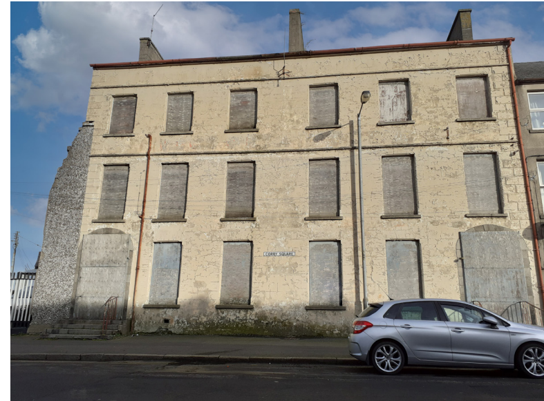
Building 1 - Listed Building
