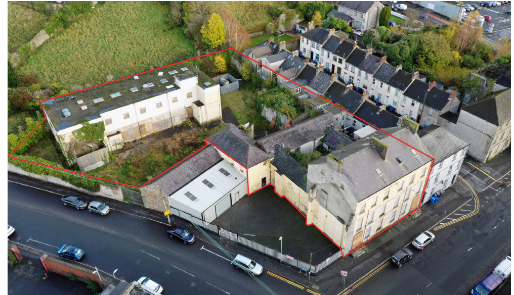
Site Side View
