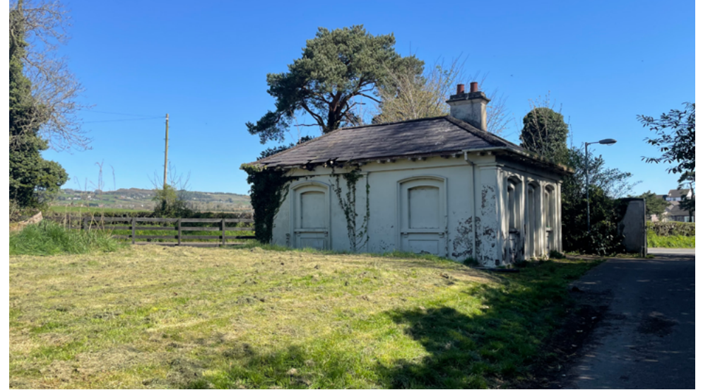
Gatehouse on Ballinderry Road
