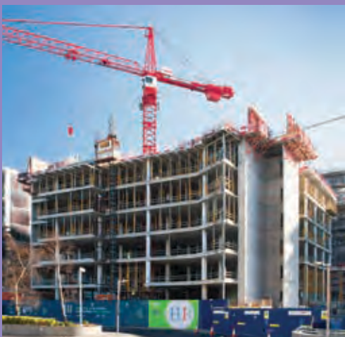
BELOW: Block H Central Park Currently under construction in the south suburbs.
