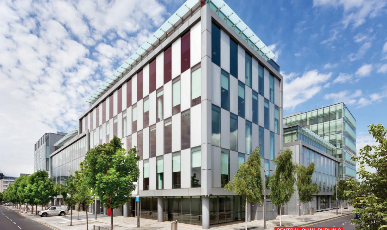
CENTRAL QUAY, DUBLIN 2
