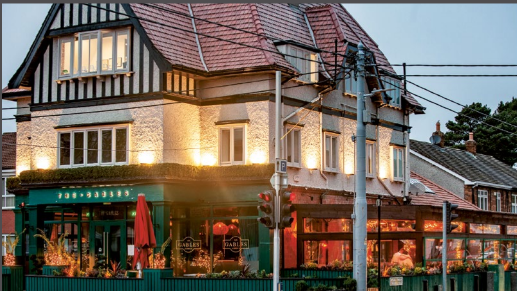
The Gables, Foxrock, Co. Dublin
