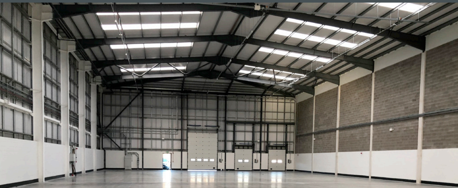
A6B NORTH CITY BUSINESS PARK, FINGLAS, DUBLIN II
