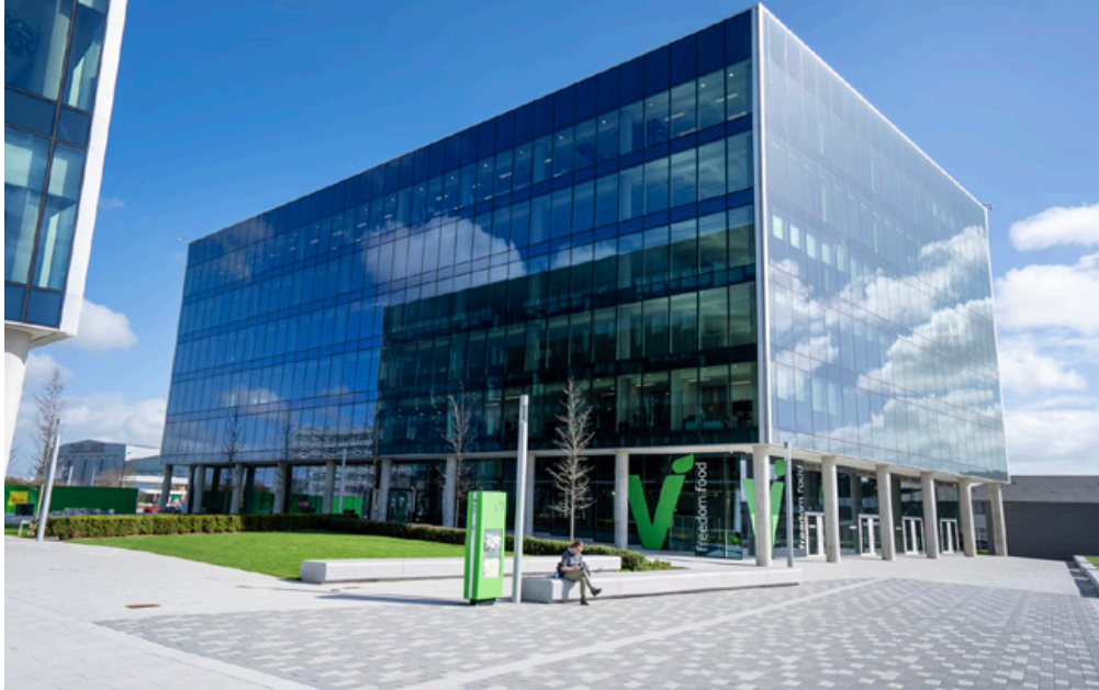
Two Dublin Airport Central, Dublin 9
