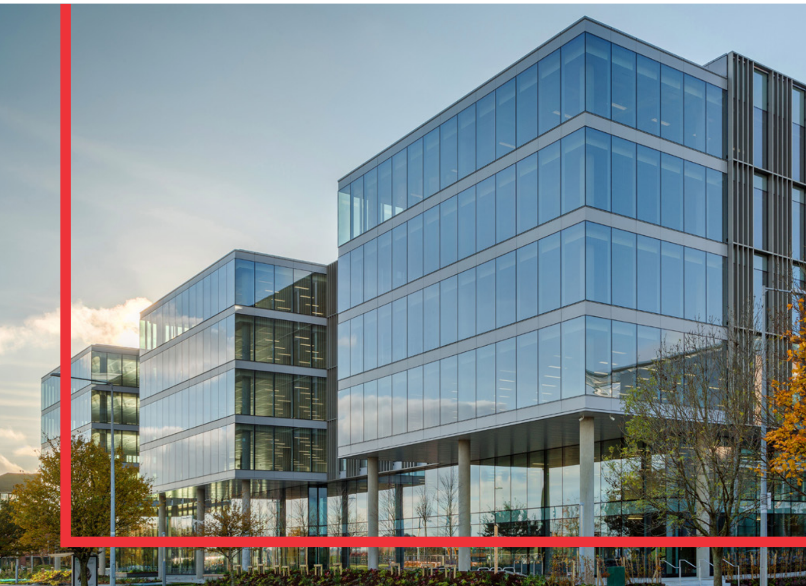
ABOVE: Termini, 3 Arkle Road, Sandyford, Dublin 18
