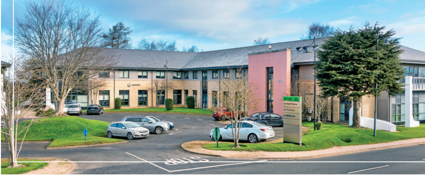
3016-3018 Lake Drive, Citywest Business Campus, Dublin 24
