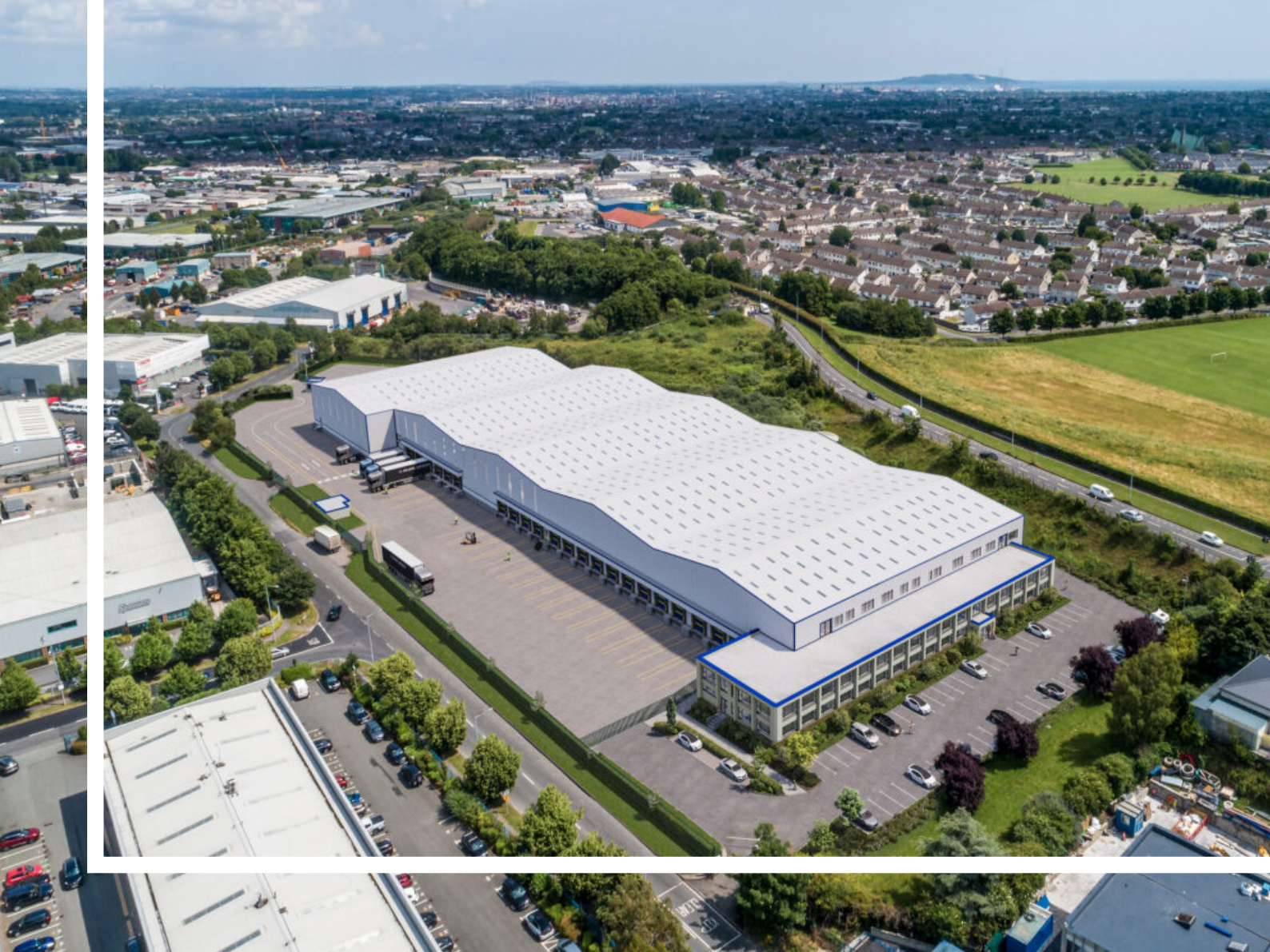
ABOVE: Ballymount Logistics Hub, Dublin 12
