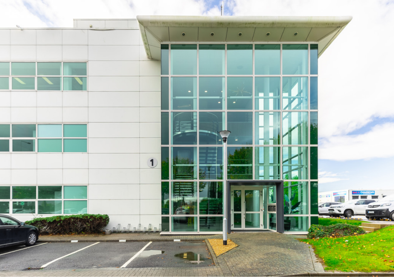
Cobalt House One, Blanchardstown Corporate Park, Dublin 15
